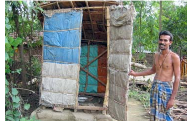
ABOVE Use of bamboo and plastics in making the super structure while the sub structure is strong and perfect. Vidyasagar colony, Kalyani, West Bengal India.
