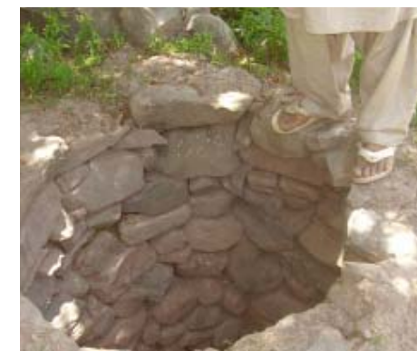
ABOVE Stones used in lining the soak pit. Photo: Syed Shah Nasir Khisro, IRSP, Mardan, NWFP, Pakistan.
